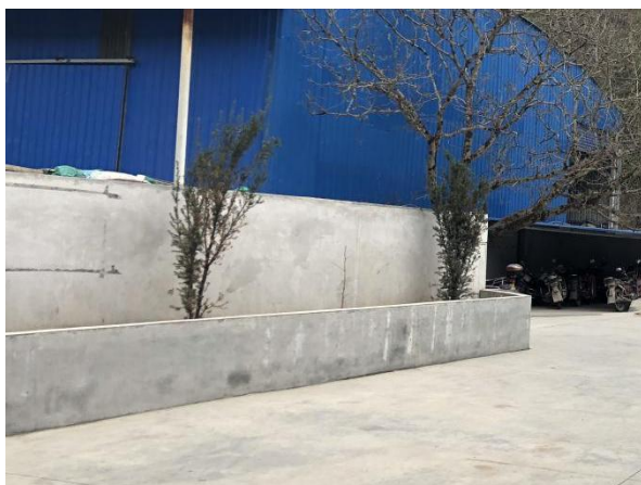
废石中转场上部西侧挡墙
